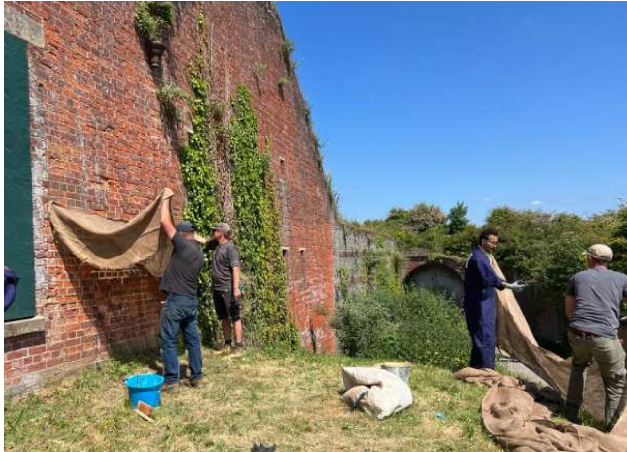
Image 5: Trainees learning how to protect the newly applied mortar. Photograph: ©DenizBeck
