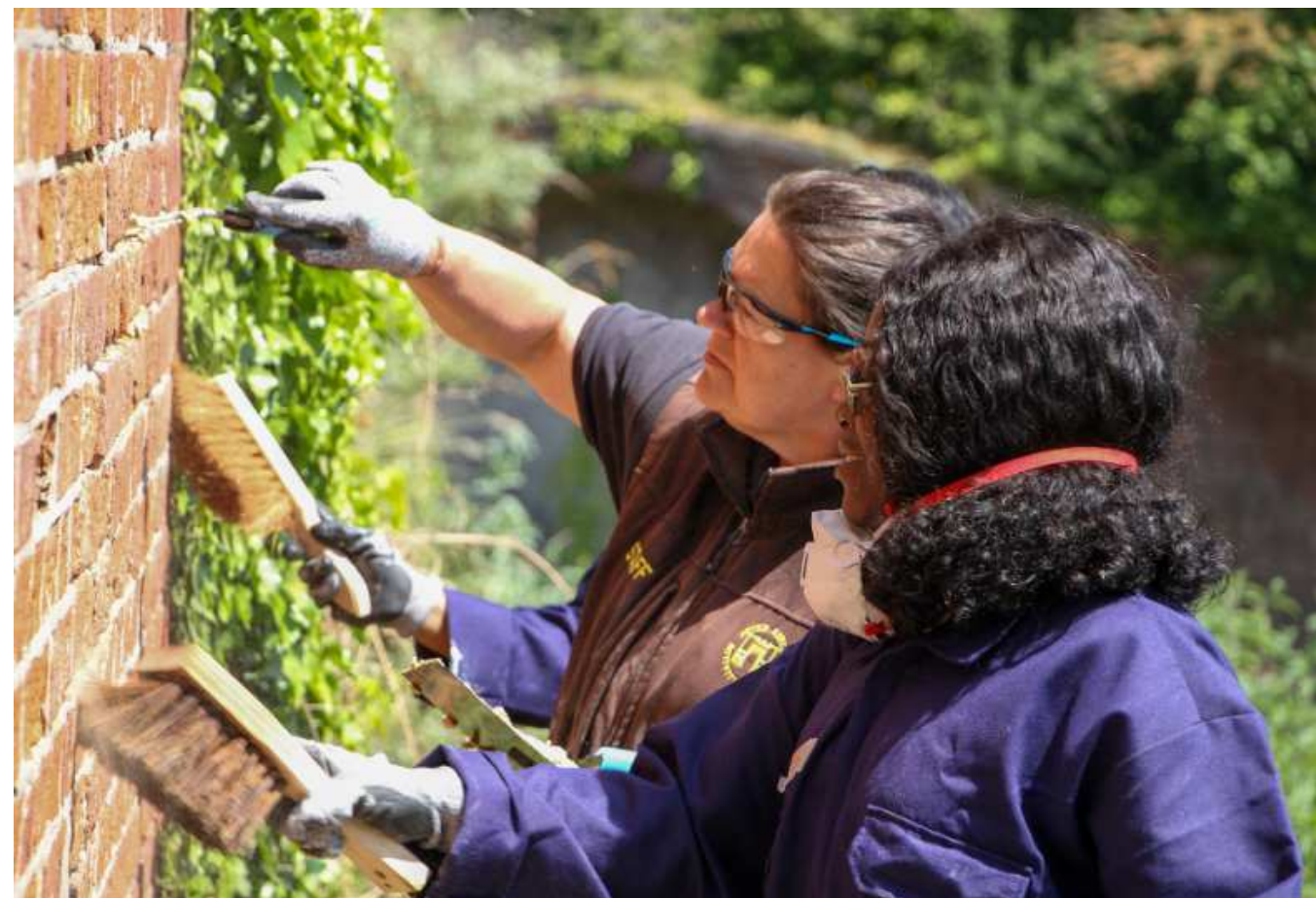
Image 3: Trailblazing women in conservation: female trainees meticulously restoring brickwork wall mortar with precision and passion. Photograph: ©SamBrooks
